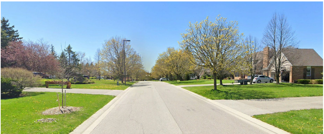
Figure 4.12: Typical Road Cross Section (Cam Fella Blvd): 10 metre local road consisting of pavement and no boulevard or sidewalk.
