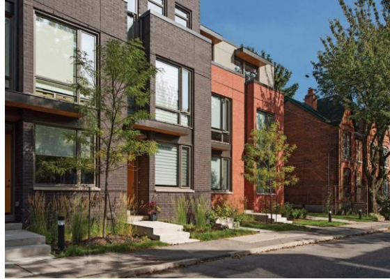
Low-rise buildings abutting heritage character area
