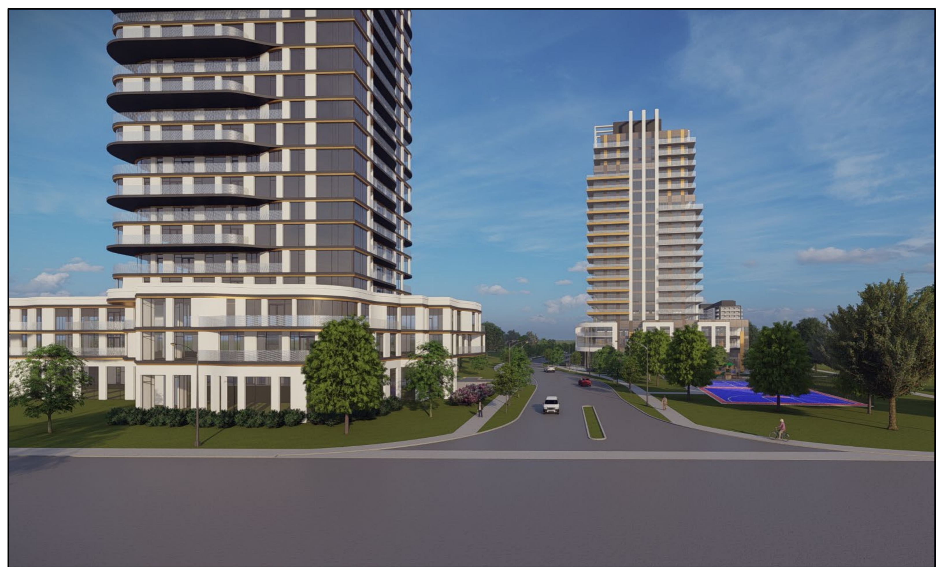
Intersection of Street A and Main Street
