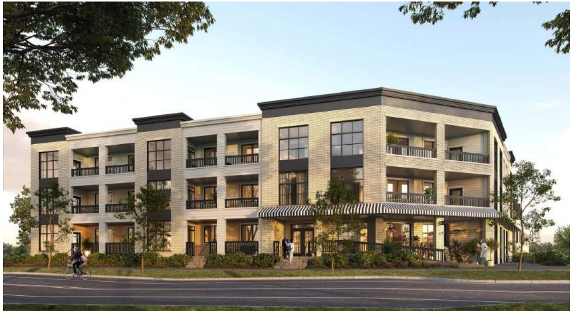
Figure 28 - Mixed-use building with retail at grade
