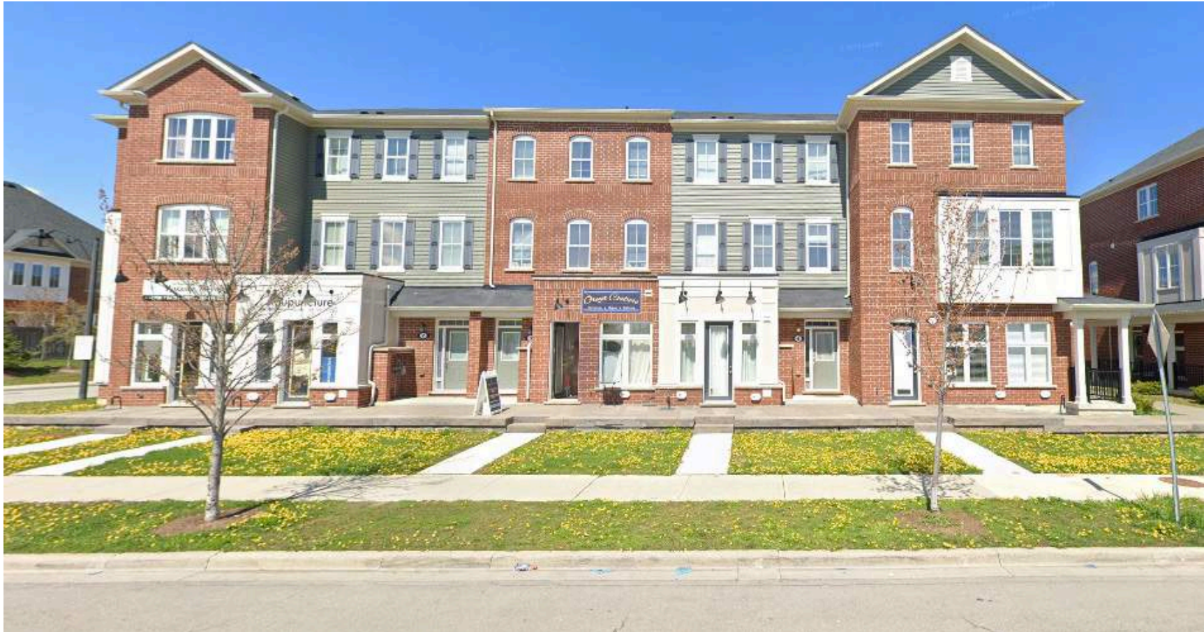
Figure 27 - Live-Work townhouse units with signage and light treatment
